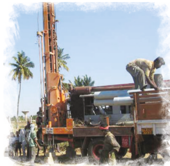
A borewell being erected
